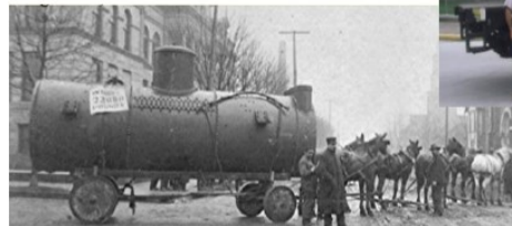
Original 22,000 lb. Courthouse Boiler (below)
