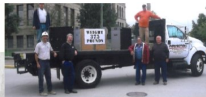
New 375 lb. Courthouse Boiler (above)
